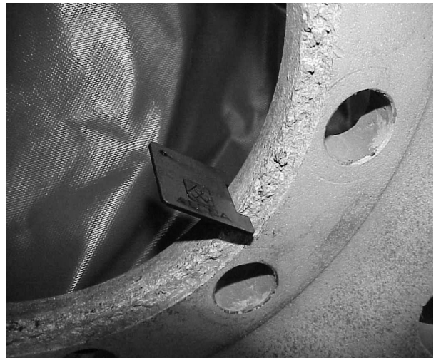
Hub bore gauge with severe corrosion. Remove any severely corroded wheel from service
